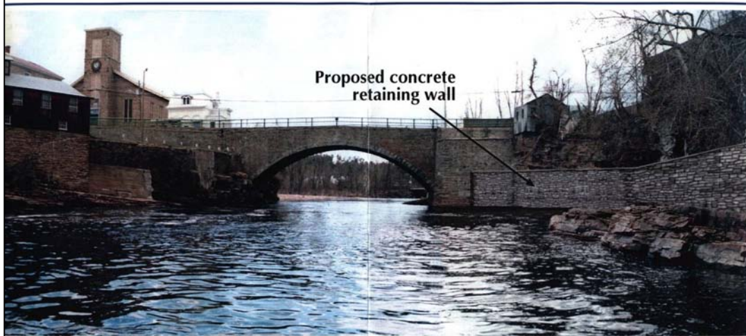
Simulation of Proposed Concrete Retaining Wall
